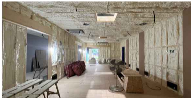
Figure 8. Construction and insulation
